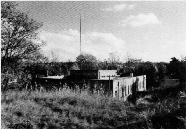
The training centre prior to demolition c.1991. The control centre is beneath this building.
